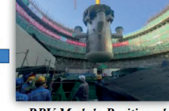
RPV Module Positioned August 10, 2023
