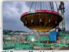
CV Bottom Head in place October 24, 2021
