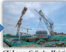
CV Lower Cylinder Hoisting February 26, 2022
